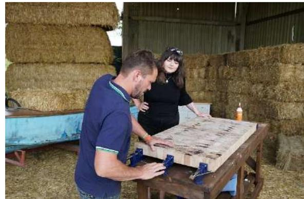
When clamping, try to keep the strips level. Expect a little movement as pressure is applied, the wood strips can be tapped back into place with a hammer.
