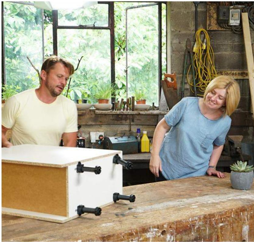
Without a worktop above it, the top of a kitchen cabinet is normally open. This will need to be filled with our section of sheet material. You will need to be able to control the flow of warm air through the cabinet, so this top will also hold the louvre vent.
