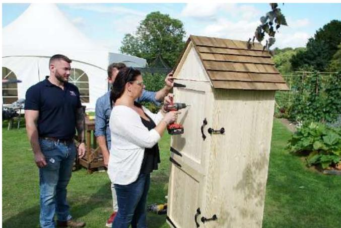
Drill a hole in the door, to take the BBQ thermometer. This will give you an idea of the heat within the smoke house.
