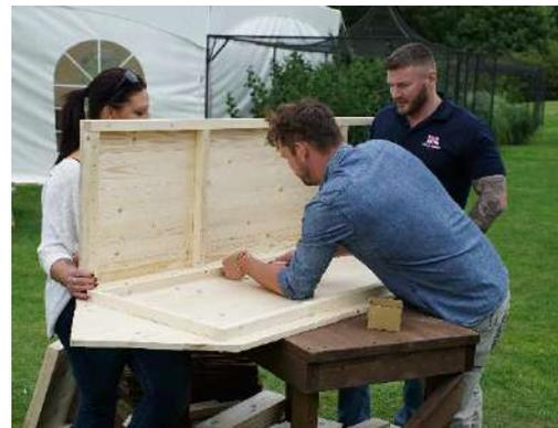
A simple frame and panels are made from the tongue and groove planks. These are all screwed together.
