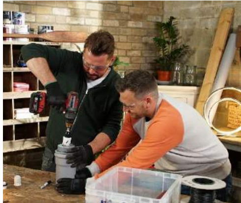
Cut a hole for the plumbing fittings to fit through.
