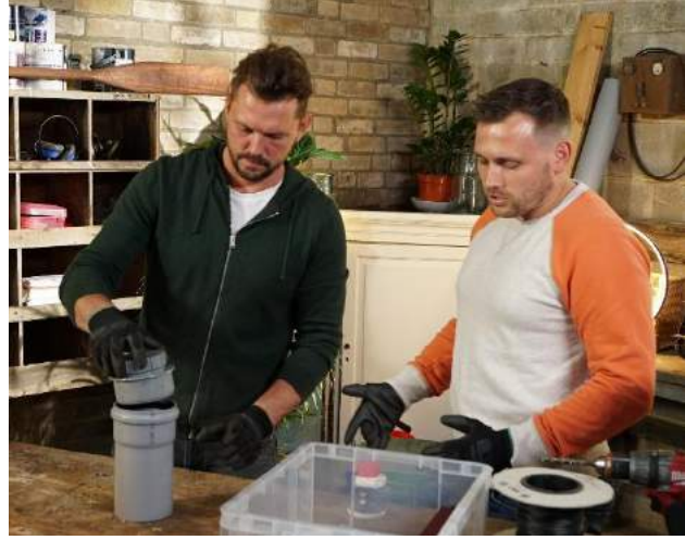
Glue the screw access hole into the drain pipe.
